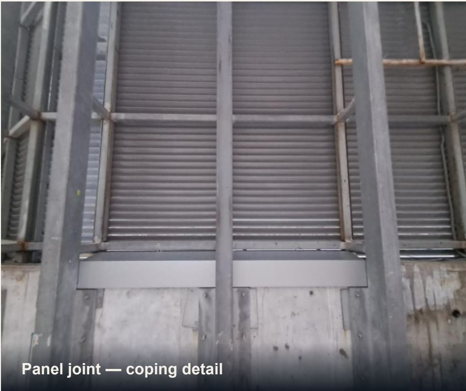
ACP substructure & insulation
